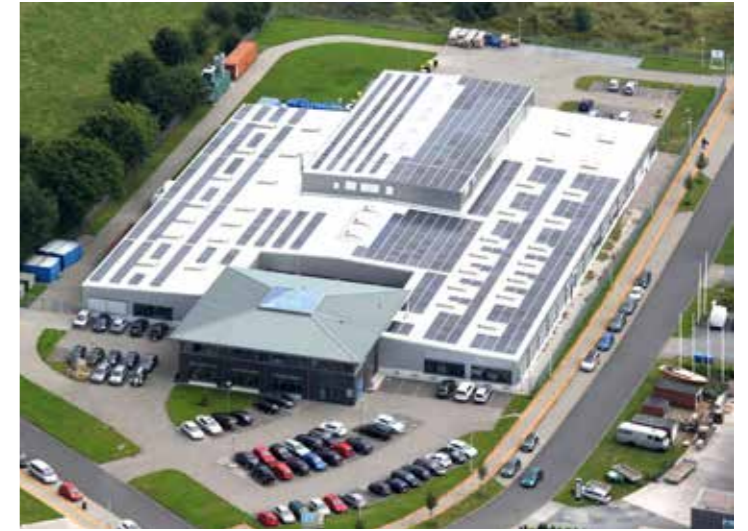
By the end of 2024, 11 industrial sites were equipped with photovoltaic power plants for self-consumption, including the Husum site in Germany.
