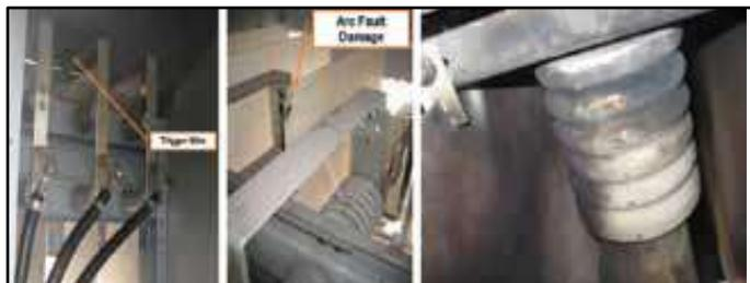
Figure 1. Trigger Wire Location (l). Damage with Current Limiting Fuses (m). Damage at 96 ms (r)
