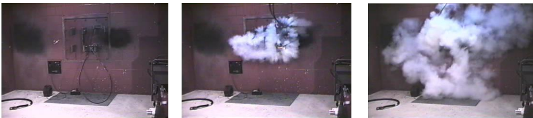
Figure 1-5. Cable damage caused by a short circuit of 35kA within 2 cycles.
