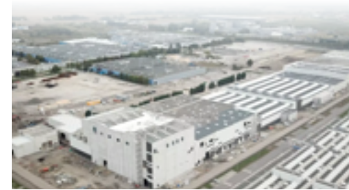
ACC gigafactory in Douvrin.
