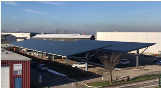
Solar power plant at Saint-Bonnet-de-Mur, France
